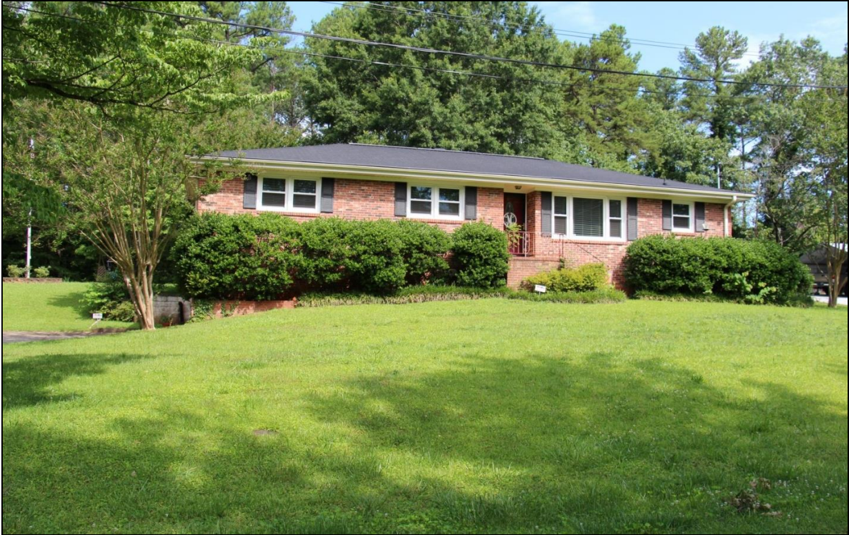
Figure 14. Ranch House with Modern Replacement Windows, Maple Circle, View Northwest
